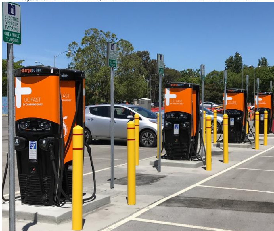
Figure 7. Eight DC Fast Chargers Installed at the NASA Ames Visitor Center Parking Lot
